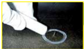
1 Location of the penetration from the inside.
